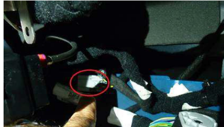
Roof Upfit Electrical Connector
